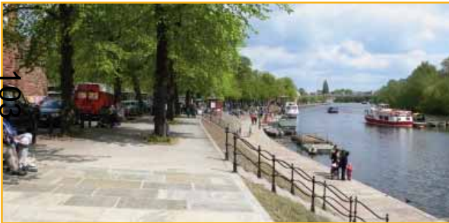
A tiered approach to the river bank, allows for an attractive riverside public realm and public space
